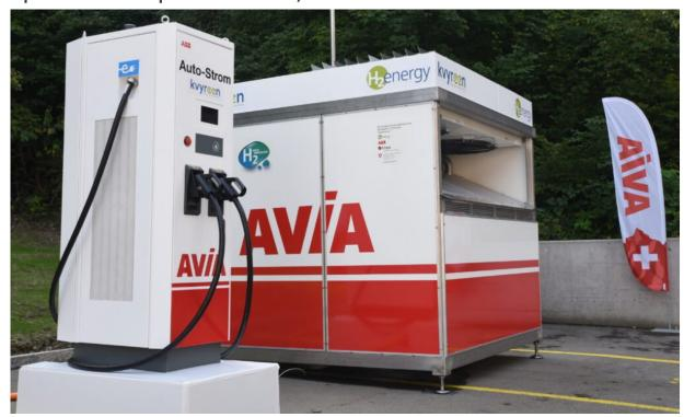
In pilot operation, the charging capacity of the system amounts to 60 kilowatts. In the later commercial application, the system will be operated with a charging capacity of up to 150 kilowatts per vehicle.
