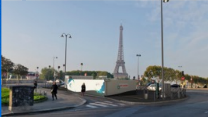
One temporary station inaugurated on December, 7th
