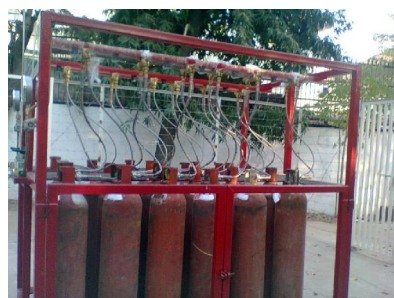
↑ Bank of Hydrogen cylinders
