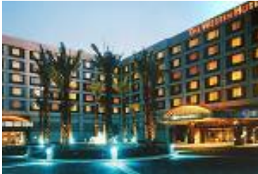
Weston at SFO Airport Nat Gas CHP
