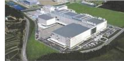
Sharp Mfg Plant Nat Gas Fuel Cell and Solar Power
